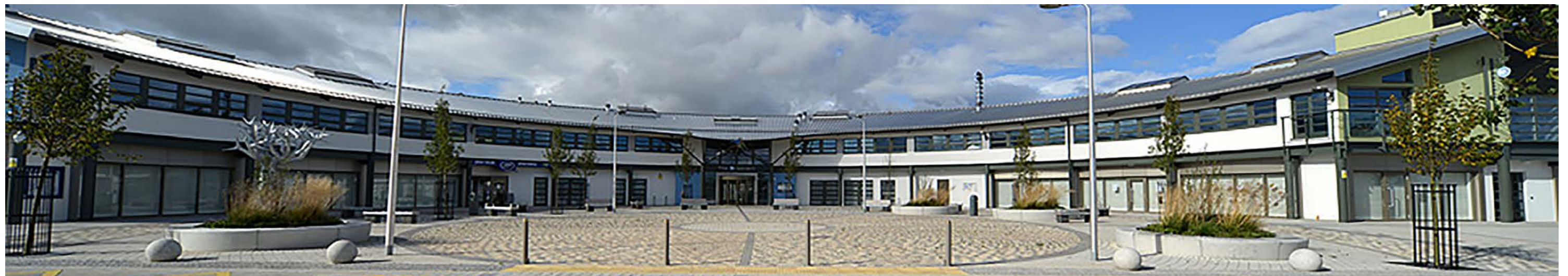
Figure 30: Sketch of the newly completed Crescent building. Source: Dundee City Council.
