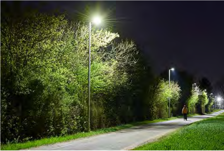
Figure 4-28 - An example of Typical Street Lighting 15
