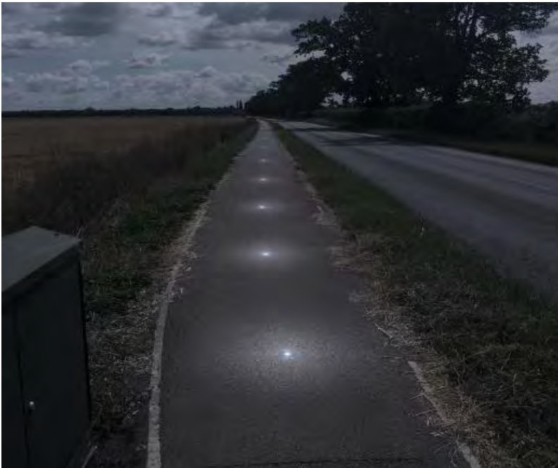
Figure 4-26 - An example of Street Lighting at footway level 13
