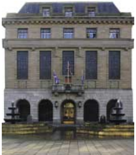
The Council Chambers Entrance as it is today
