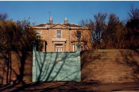
Boundary walls come in different shapes, forms, heights and materials. In Dundee walls might be brick or rendered block, but in conservation areas they are commonly of local sandstone. The stone could be ashlar blocks (square-edged dressed stones) or of random rubble (unshaped stones). Although many walls are pointed with a cement mortar, the appropriate and historic mortar for stone is lime.
