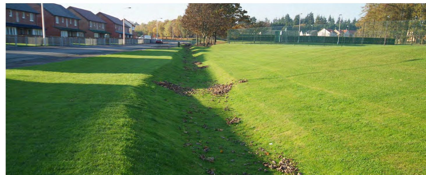
Figure 22: Above are examples of established, attractive and successful SUDS in Ardler, Dundee.
