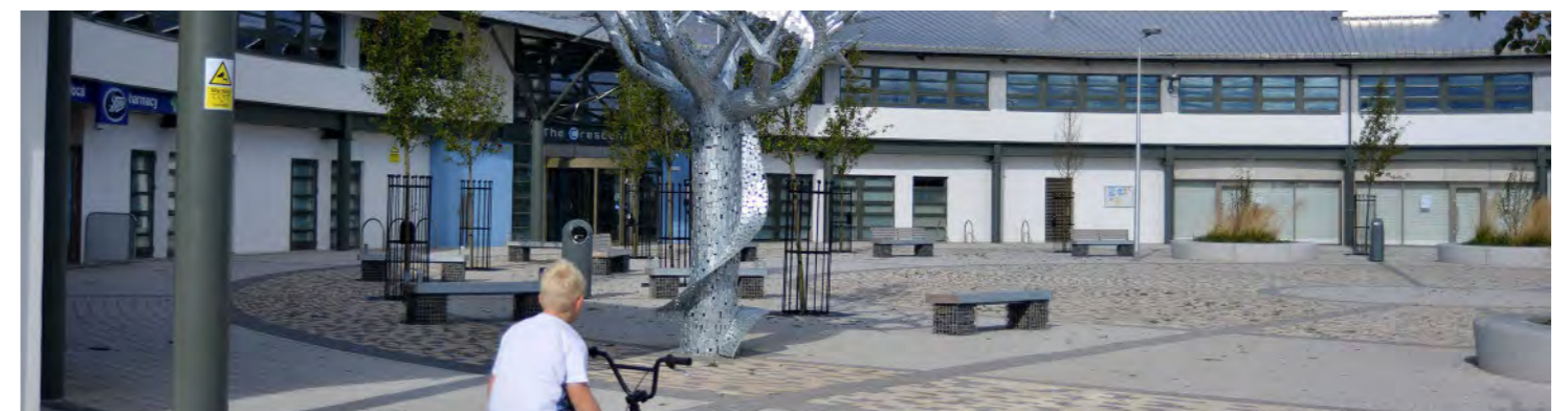
Figure 05: Examples of new developments in Whitfield. From top to bottom: Summerfield Crescent and The Crescent (life services building) on Lothian Crescent.
